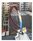
On construction sites, the Air Heater is also often used as second heating unit by our customers. For example, when the larger main line is cured with one of our steam generators, smaller secondary lines or drain pipes can be heated and cured with the Air Heater. By means of this technique our Air Heater has more than paid off even after a short time and you will never want to do without it again.
